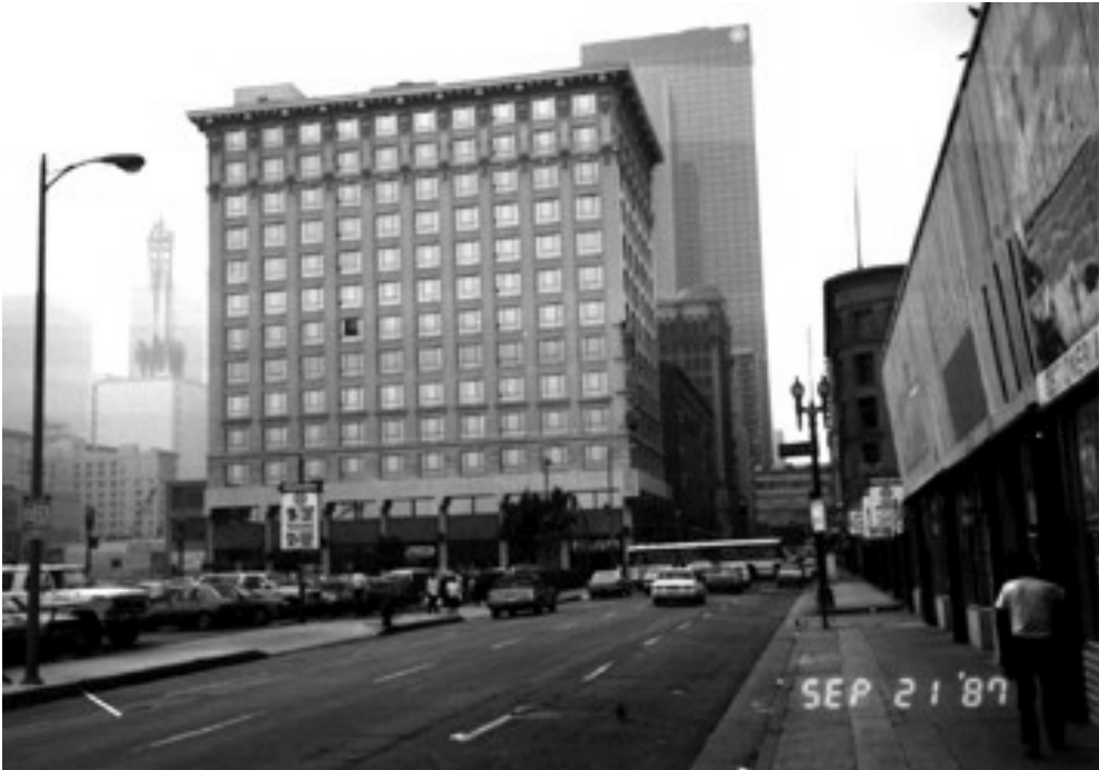
Figure 1. Photo of thirteen-story instrumented building (source: http://www.strongmotioncenter.org/cgi-bin/CESMD/stationhtml.pl?stationID=CE24567&network=CGS ).
